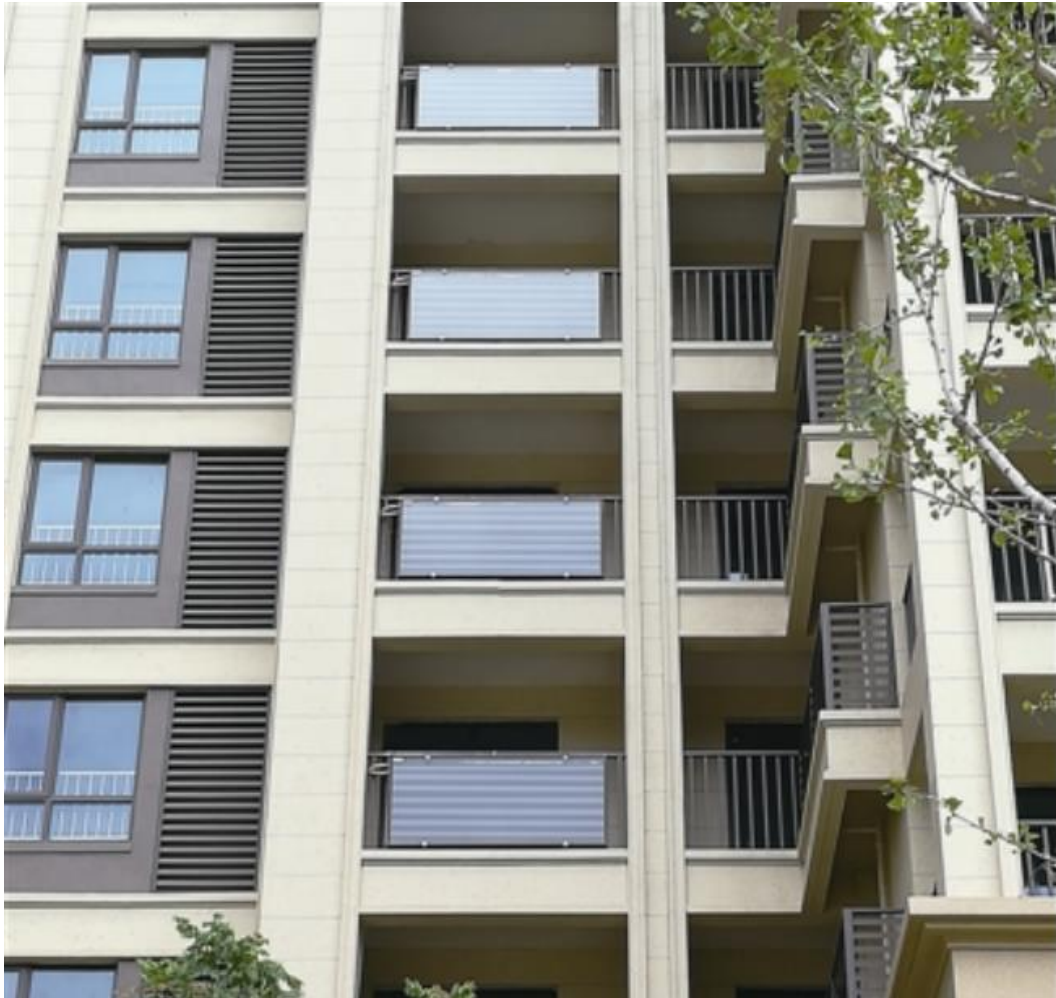
Figure 2 – Curved surface heat absorption solar water heater
