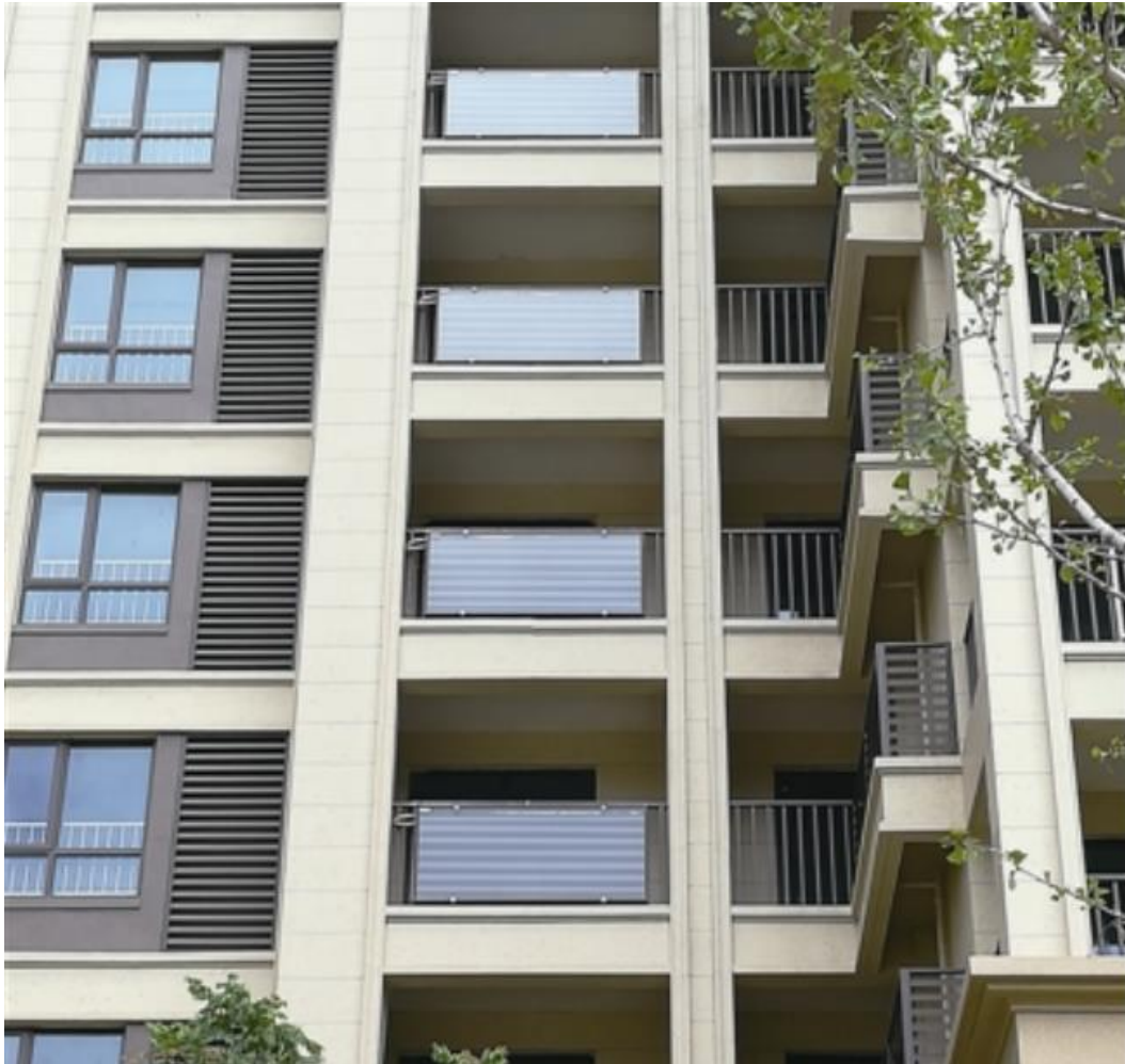
Figure 2 – Curved surface heat absorption solar water heater
