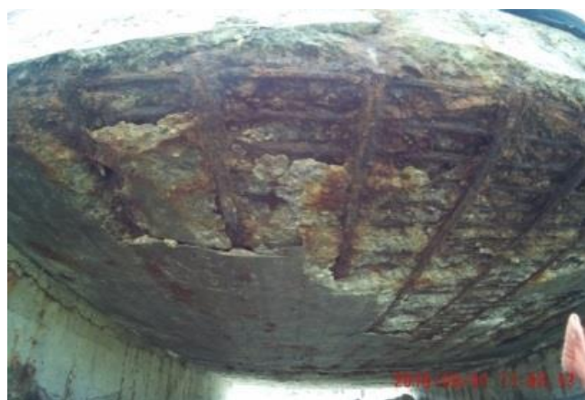
Figure 5 – Span of the pedestrian bridge of the Kholmok sea trade port
