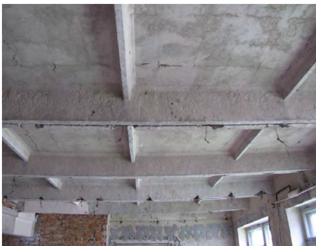
Figure 1 – General view of the evaluated ribbed slabs
